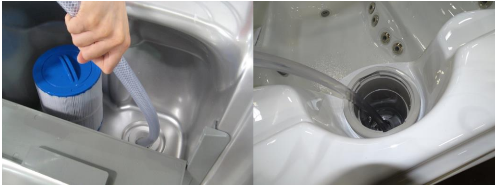
Figure 8. Filling Location in Filter Housing
