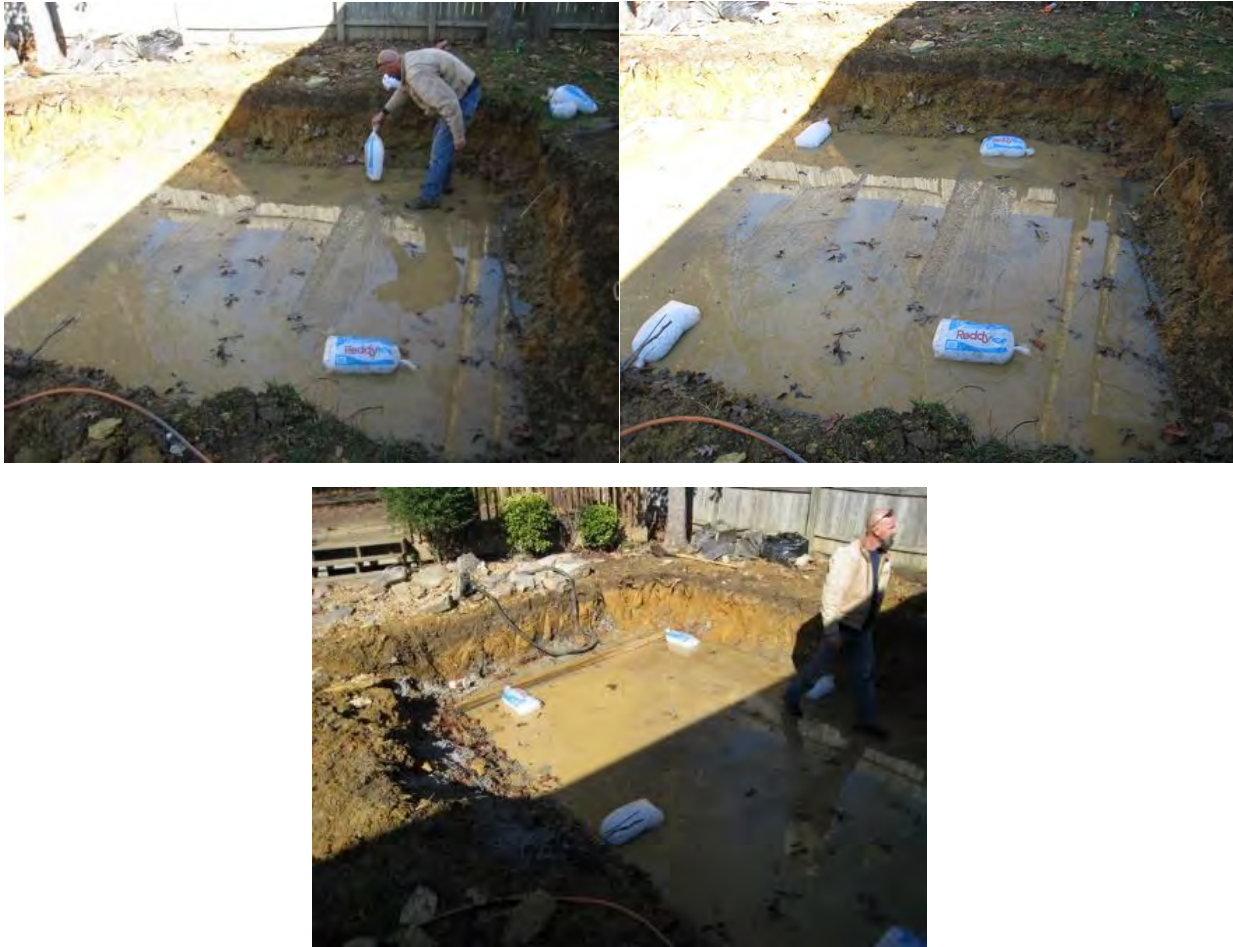
Figure 7. Ice Bag Positioning in Excavation
