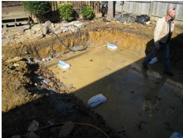
Figure 7. Ice Bag Positioning in Excavation
