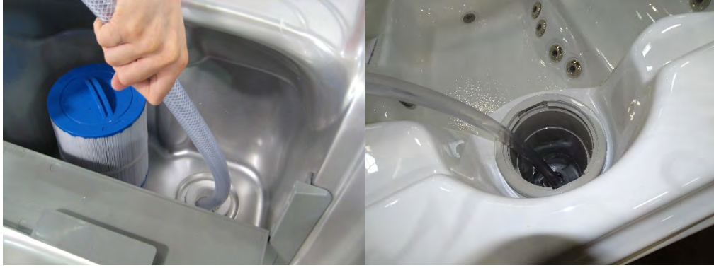
Figure 7. Filling Location in Filter Housing
